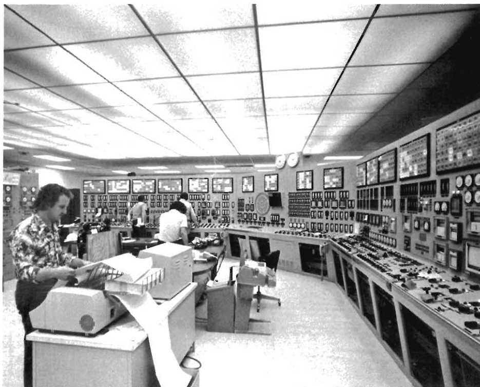
Fig. 6. Control room of a commercial nuclear power plant. A myriad of lights, dials, and switches monitors and controls all the complex systems within the plant. (Photo courtesy of Florida Power & Light Company.)
