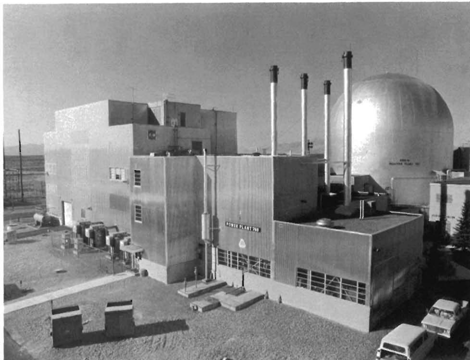
Fig. 13. The EBR-II reactor is located at Idaho National Engineering Laboratory near Idaho Falls, Idaho. This liquid-metal-cooled fast breeder reactor has operated successfully for over 15 years. The reactor produces up to 20 megawatts of electrical energy and has had an excellent history of reliable operation. A predecessor of EBR-II, a small reactor called EBR-I, produced the first nuclear-generated electricity in 1951. (Photo courtesy of Argonne National Laboratory.)
